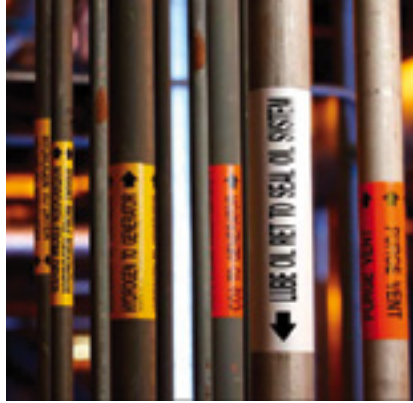
8. Label adhesion is prone to failure under extreme plant conditions (above)
