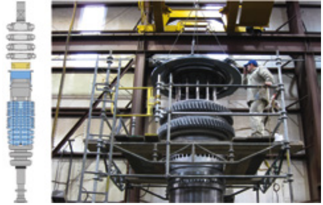
4. Turbine wheels are removed individually
