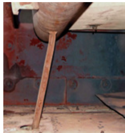
2. Differential expansion amplifies drain lateral displacement
