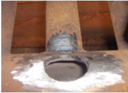
10, 11. Old tube section removed, header hole is cleaned up (left) before dutchman is welded in (right)
