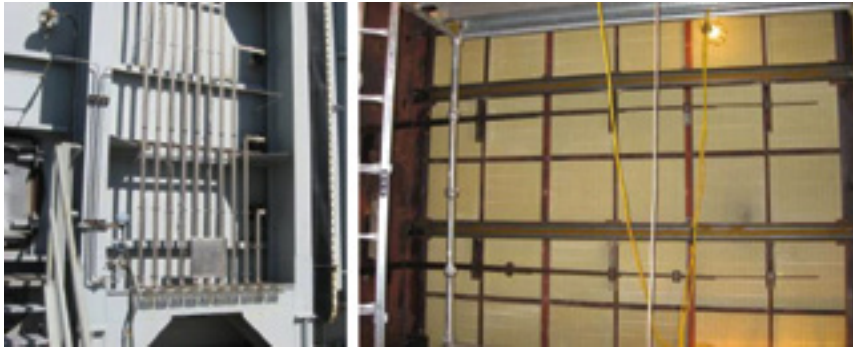
5. Permanent sample-probe grid can be located outside the duct (left) or inside (right)
