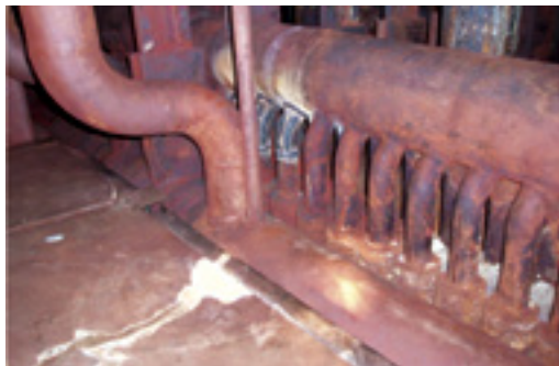
12. Plugging of tube through header should be the solution of last resort
