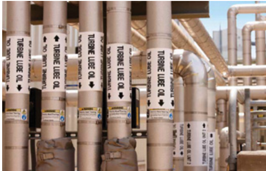
10. Wrap-around labels ensure identification from all sides
