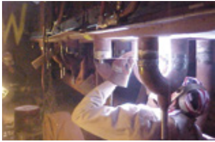
6, 7. Jumper piping is cut (left) to allow raising of the panel at right for tube repair
