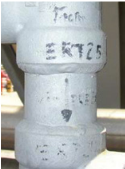
2. Ink marking on piping , an expedient for plant staff, often becomes the permanent label (right)
