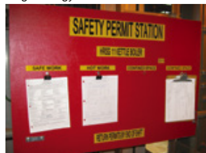
Safety permit stations are strategically located on the deck plates. They are easily accessible and highly visible. Granite Ridge Energy
