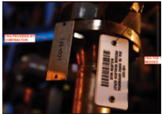
11, 12. The tag will stay with the foundation, but what does it say? (left) The more information, the better (right)
