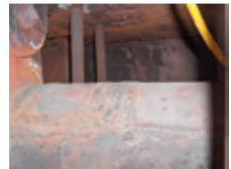
13-15. Good header patch (no sharp corners) is at left, bad patch with squared-off corners is in center, ugly patches with square corners are at right
