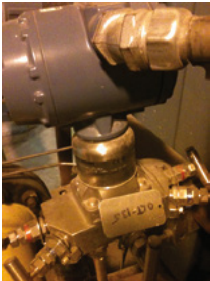
6. Without plant specifications, labels may vary greatly and have inadequate information and non-durable inscriptions (left)
