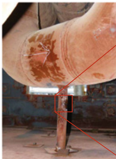
3. Drains that collide with the floor liner or casing often suffer stress-induced cracking
