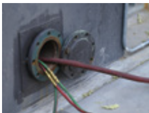
Penetrations on enclosures eliminate the need to run lines, cords, and leads through doorways. Walter M Higgins Generating Station
