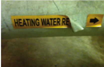
8. Label adhesion is prone to failure under extreme plant conditions (above)
