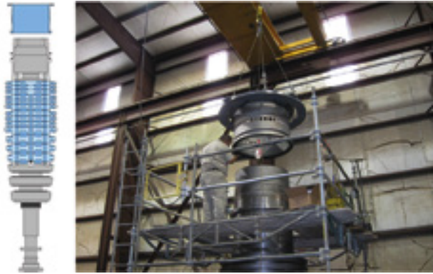
5. Air-separator sleeve is removed to access compressor through bolts
