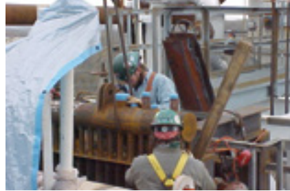
6, 7. Jumper piping is cut (left) to allow raising of the panel at right for tube repair
