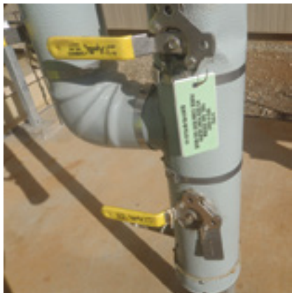
1. Effective tags clearly identify equipment (above)
