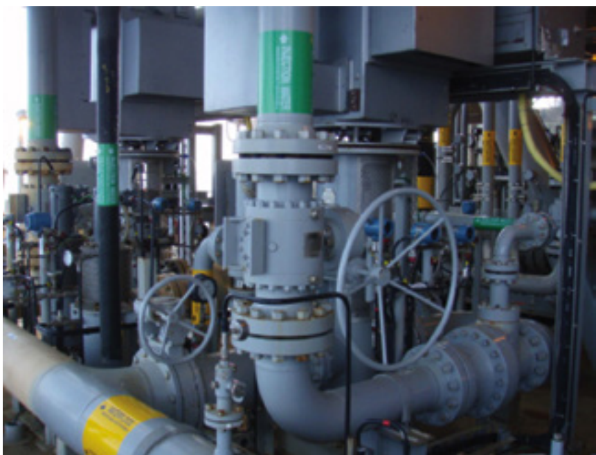
3. Good label placement requires attention to detail to ensure visibility
