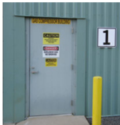
Highly visible numbers (18 × 18 in.) at all key entrances to plant save time in directing emergency response units to the proper location. The numbers should be high enough off the ground that the line of sight cannot be blocked by deliveries, parked vehicles, etc. Granite Ridge Energy
