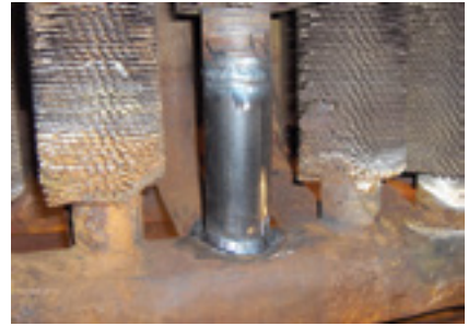
10, 11. Old tube section removed, header hole is cleaned up (left) before dutchman is welded in (right)
