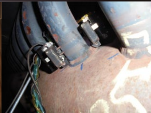
Tube to Header Weld Examination for Cracking
