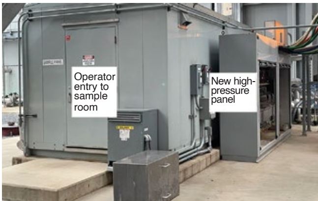
1. Relocating the sample panel eliminated concerns associated with having high-pressure/high-temperature fluid in the space-confined sample room
