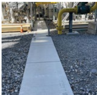
11. A plant-wide system of concrete walkways was designed and installed to avoid the slips, falls, and ankle injuries associated with traversing areas "finished" with crushed rock
