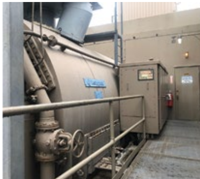
2. New H 2 purge control system and dryer for a peaker (right) replaced one which had the controls cabinet (left) hanging off of the unit—just one facet of taking a gas turbine that “hardly runs” to one now running baseload
