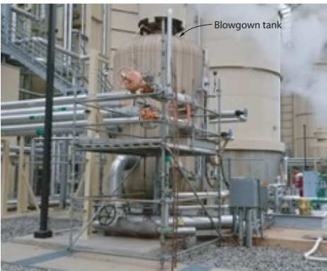
8. Temporary scaffolding was provided around HRSG blowdown tanks to access HP and IP blowdown valves (left). Permanent access was by way of guard rails fabricated around the tanks and other equipment (right)
