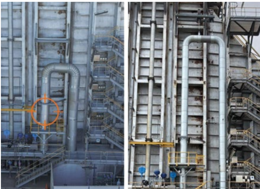
4. Spray loop redesign before (left) and after (right)
