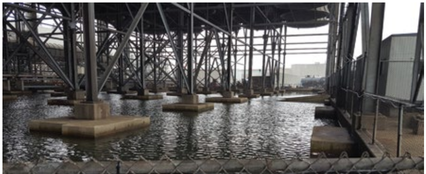
1. Linden’s storm-water detention pond is protected to the extent possible by the air-cooled condenser
