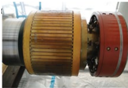
14. One of several excitation retrofits identified in the slide deck. Specs for this unit: 158 kVA, 3600 rpm, 13.8 kV, 6600 amps, 0.85 pf
