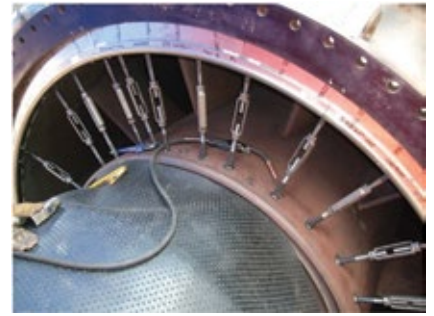
7. Flex-seal retention assembly can extend the interval between seal replacements
