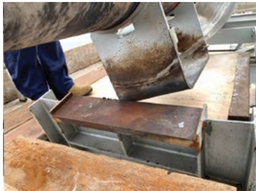
11. Main-steam slide support disengagement
