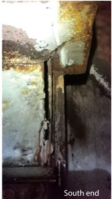
9. Vertical transition-duct joint damage. North-end metal joint cracked again within two weeks
