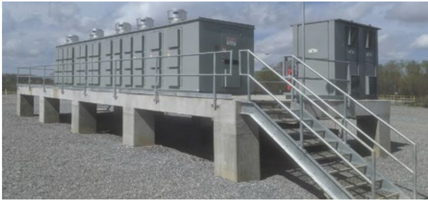
5. Harmonic filter for grounding transformer almost doubled in size after being redesigned based on actual startup data
