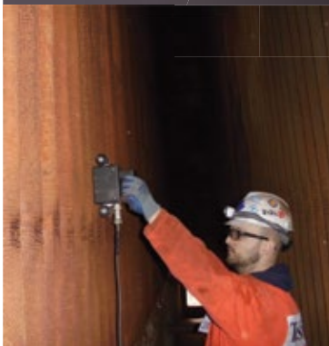
Through Fin Tube Scanning for Wall Thinning
