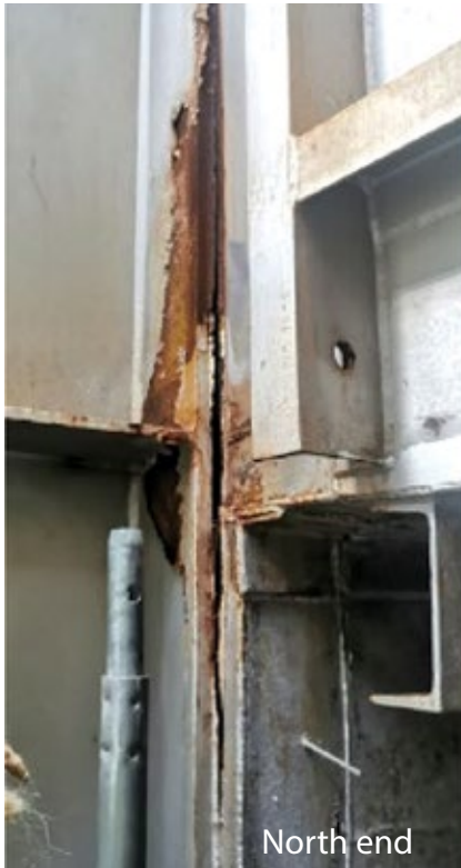
9. Vertical transition-duct joint damage. North-end metal joint cracked again within two weeks
