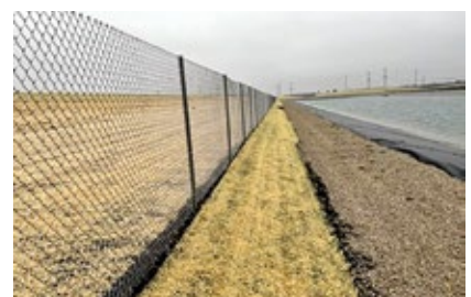
4. Fence impedes access to the pond by trespassers
