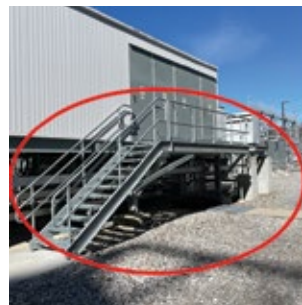
12. LCI staircases enabled operators safer access for routine equipment checks than temporary scaffolding (left). A platform for service-water cartridge filter changeouts (right) was installed to eliminate the need for step ladders
