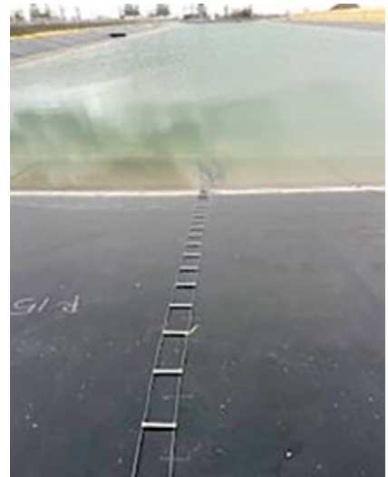
2. Ladders mounted around pond boundary facilitate escape from a potential hazard
