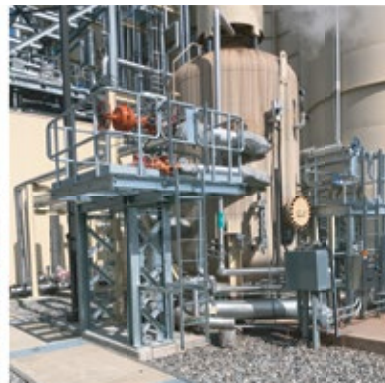
8. Temporary scaffolding was provided around HRSG blowdown tanks to access HP and IP blowdown valves (left). Permanent access was by way of guard rails fabricated around the tanks and other equipment (right)
