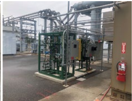
2. New H 2 purge control system and dryer for a peaker (right) replaced one which had the controls cabinet (left) hanging off of the unit—just one facet of taking a gas turbine that “hardly runs” to one now running baseload
