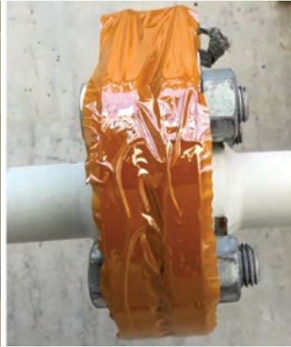
2, 3. Leading options for safety improvement include HazGas detectors for hydrogen (left) and H 2 detection tape (right)
