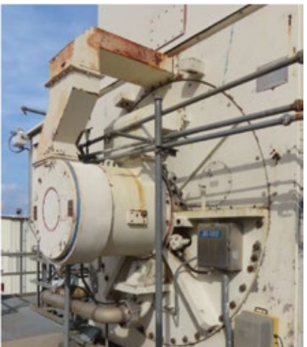
14. One of several excitation retrofits identified in the slide deck. Specs for this unit: 158 kVA, 3600 rpm, 13.8 kV, 6600 amps, 0.85 pf
