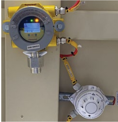
2, 3. Leading options for safety improvement include HazGas detectors for hydrogen (left) and H 2 detection tape (right)
