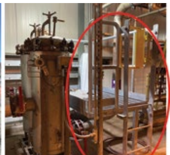
12. LCI staircases enabled operators safer access for routine equipment checks than temporary scaffolding (left). A platform for service-water cartridge filter changeouts (right) was installed to eliminate the need for step ladders
