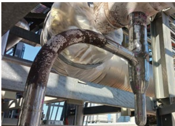
5. Drain pot with forged tee
