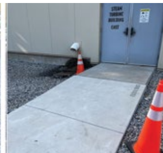
11. A plant-wide system of concrete walkways was designed and installed to avoid the slips, falls, and ankle injuries associated with traversing areas "finished" with crushed rock
