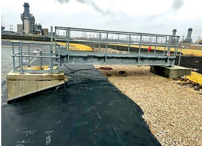
1. Walkway with handrails was installed over the pond liner
