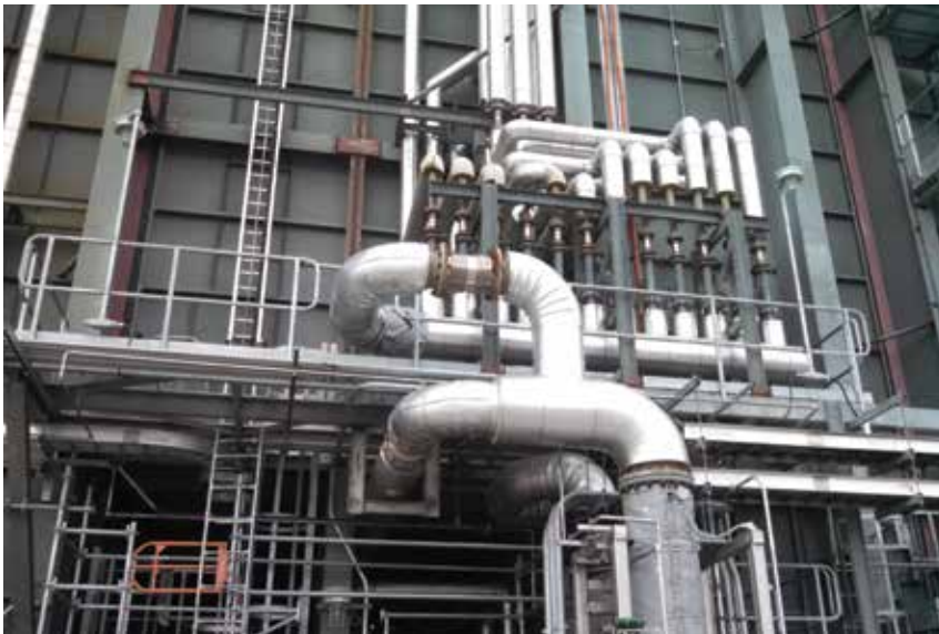
1, 2. Ammonia distribution piping to the AIG is shown at left. Control zones should be able to adjust ammonia in sections of the ductwork. Photo, right, illustrates traverse tuning which involves taking measurements of ammonia distribution at each of the eight AIG elevations. The more zones, the better the tuning capability
