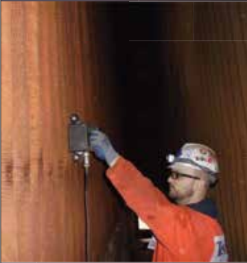
Through Fin Tube Scanning for Wall Thinning
