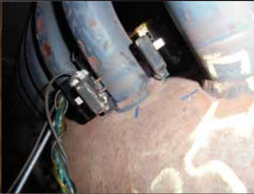
Tube to Header Weld Examination for Cracking
