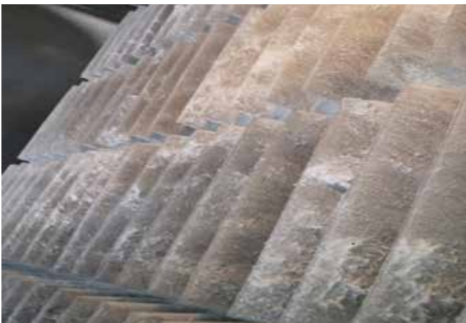
1. Snow buildup on GT-inlet prefilters is at left, snow plugging the final filter at right
