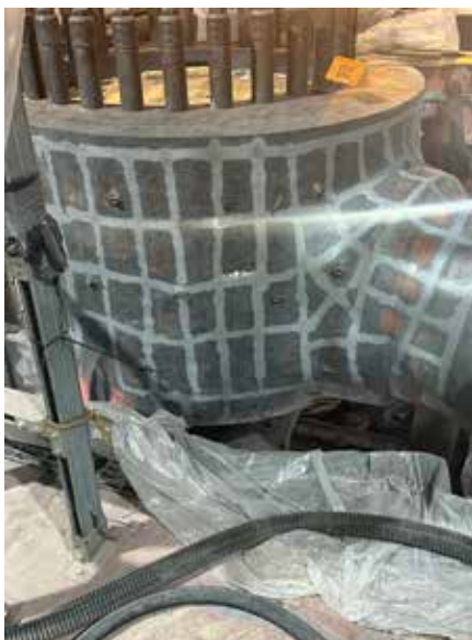
1. Planned layout of the valve warming system begins with the grid illustrated at the left. Installation of the heating coil (center) is next. Insulated valve is at right with step protection
