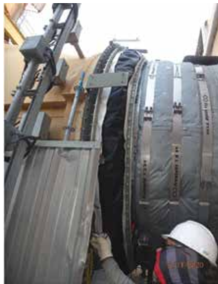
Frenzelit. Installing an upgraded expansion joint
