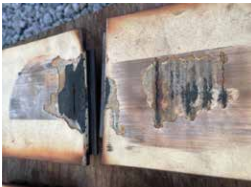
Damage to Row 1 ring segment was an emergent issue faced during unit's first HGPI
