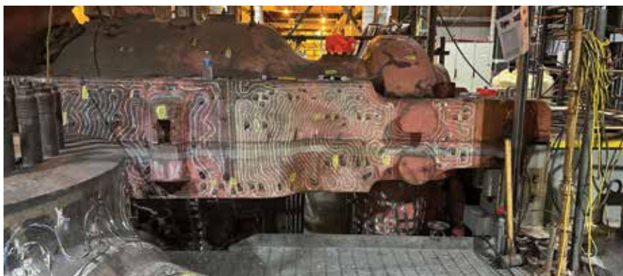
2. Heating wires installed on the steam-turbine casing at the split line
