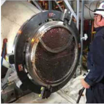
Machining the face of the tubesheet helped restore the condition of this kettle boiler
