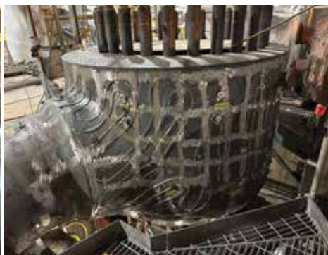
1. Planned layout of the valve warming system begins with the grid illustrated at the left. Installation of the heating coil (center) is next. Insulated valve is at right with step protection
