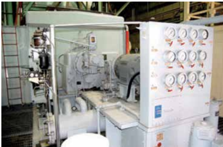
8. Accessory base contains the auxiliaries for starting and operating the gas turbine
