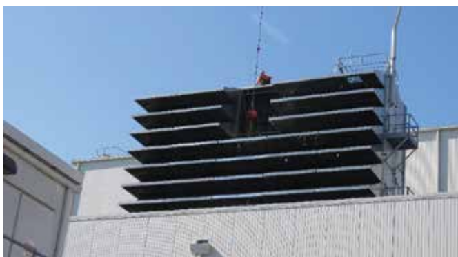
4. Snow hoods (left) were removed (right) to accommodate the anti-icing module
