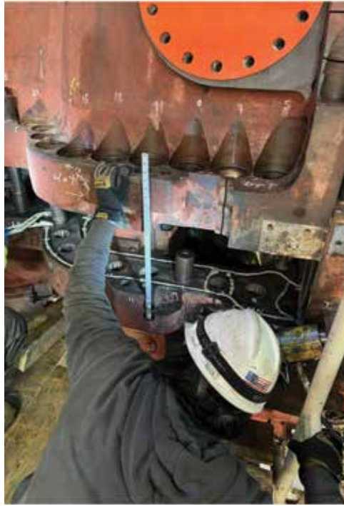
Hands-free measurement during casing lifts
