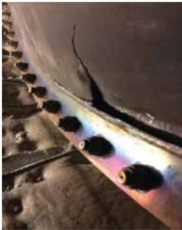
Machining the face of the tubesheet helped restore the condition of this kettle boiler
