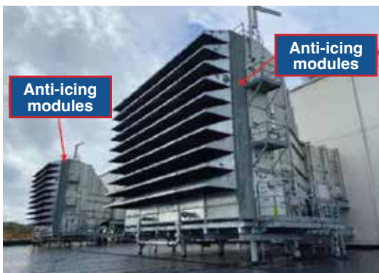
7. Anti-icing modules installed
