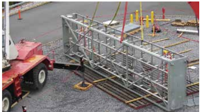
3. Anti-icing module is ready for installation
