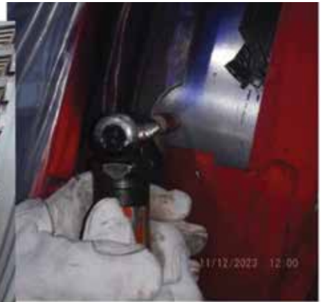
Rotor alignment was one of the challenges faced after replacing Row 3 interstage seals
