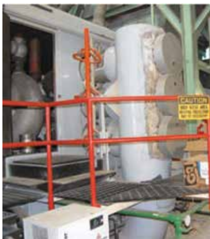
7. One combustor manifold is located on either side of the engine
