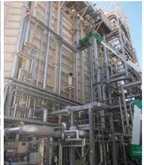
1, 2. Ammonia distribution piping to the AIG is shown at left. Control zones should be able to adjust ammonia in sections of the ductwork. Photo, right, illustrates traverse tuning which involves taking measurements of ammonia distribution at each of the eight AIG elevations. The more zones, the better the tuning capability
