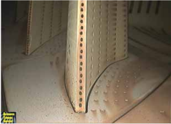
Advanced first-stage vanes in GTOP system remain pristine after two years of service
