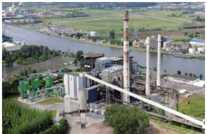
6. Engie Electrobél coal-fired station went into service in 1979
