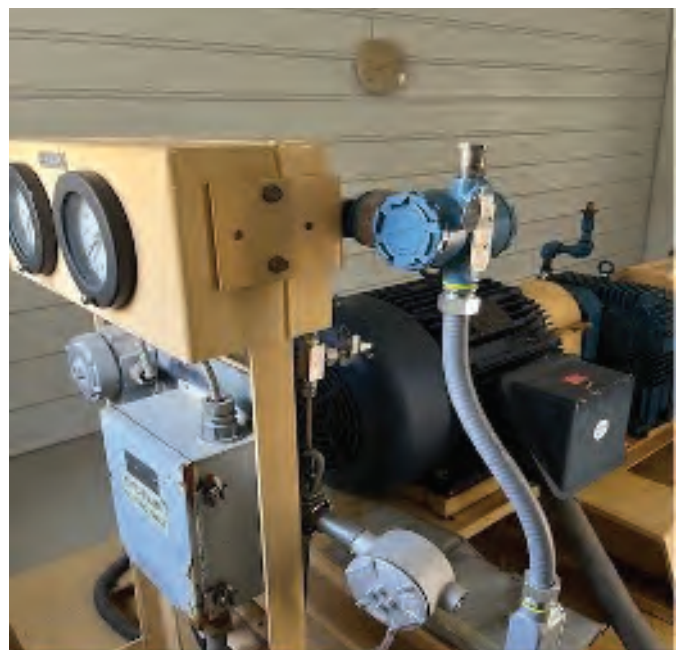
NOx-water pressure transmitter was relocated to protect against freeze-up
