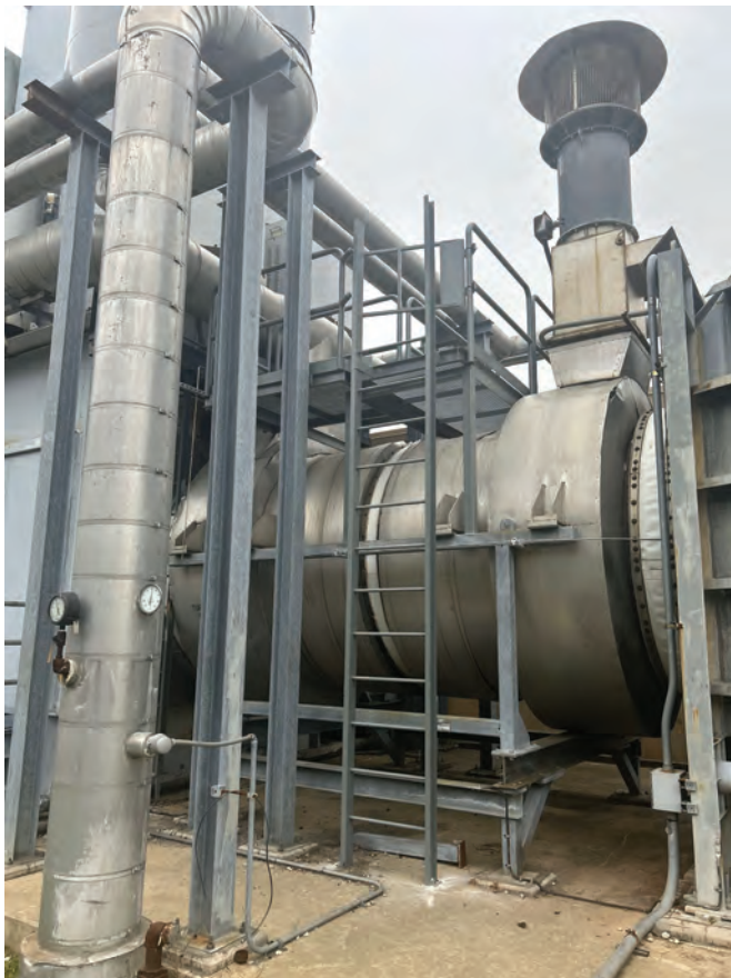
Ladder and work platform, a safety initiative, were mounted on the gas-turbine exhaust section (left). Platform provides direct access to the blower fan and motor for maintenance (right)
