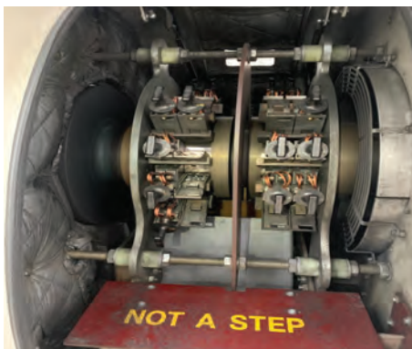
7. GE brush rigging supplied with the generator was realigned multiple times to mitigate cracking (left) but that proved unsuccessful. Success was achieved by truing the rings and installing a Cutsforth EASYchange Brush System (right)
