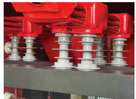
8. With Crown-sulators in place, switchgear has better mechanical bracing and dewpoint-rated hi-pot withstand
