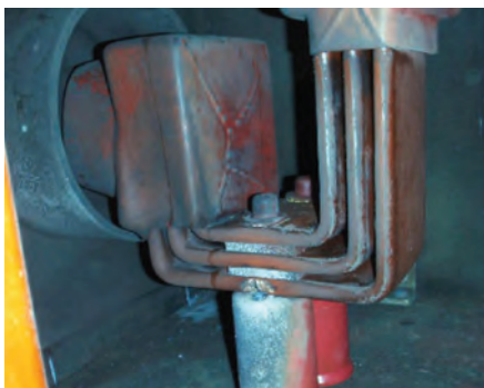
7. Glastic stand-offs used in many of the original cells were replaced with more durable Crown-sulators
