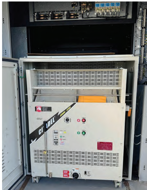
12. Citadel draw-out breaker is introduced to the GAC and its one-high enclosure
