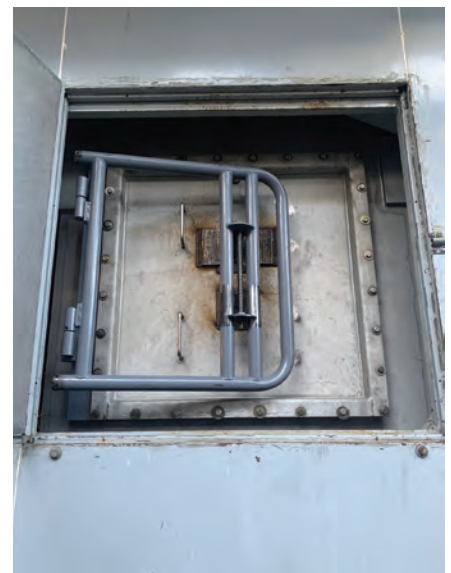
FOD-screen inspection door before addition of handle and hinge (left). After several years of manually removing the door, personnel began using a hook and pulley system to lower the door. While safer, the task still presented a moderate risk of injury to staff if not properly planned and executed. Contractors install pre-fabricated handle and hinge assembly in center photo. Finished product is at right
