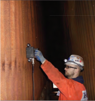
Through Fin Tube Scanning for Wall Thinning
