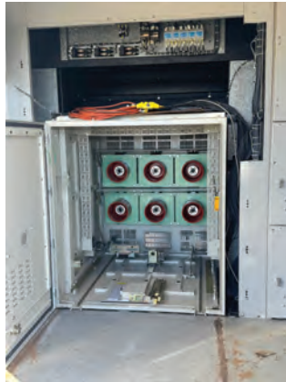
9. Citadel cell is lifted into the space formerly occupied by the original cell
