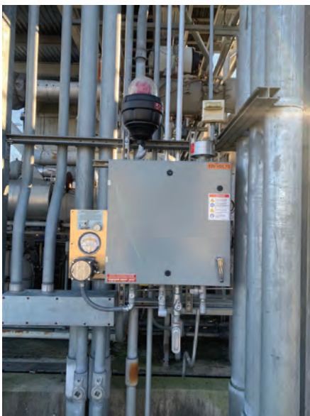
Wireless position monitor (left) is installed on one of the gas-compressor discharge headers; pressurized enclosure cabinet at right contains the wireless gateway and Modbus interface
