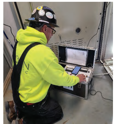
13. Testing and operational checks confirm retrofill is ready for service
