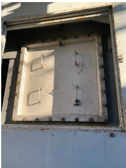
FOD-screen inspection door before addition of handle and hinge (left). After several years of manually removing the door, personnel began using a hook and pulley system to lower the door. While safer, the task still presented a moderate risk of injury to staff if not properly planned and executed. Contractors install pre-fabricated handle and hinge assembly in center photo. Finished product is at right
