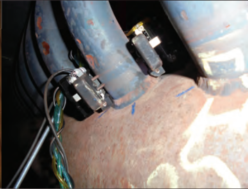
Tube to Header Weld Examination for Cracking
