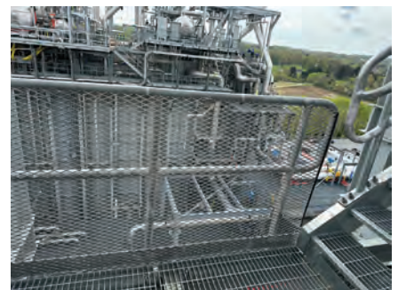
5. Landing zone (top) safety mod features an expanded metal barricade (bottom) to prevent objects from falling off the catwalk
