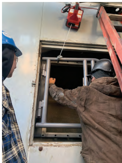
FOD-screen inspection door before addition of handle and hinge (left). After several years of manually removing the door, personnel began using a hook and pulley system to lower the door. While safer, the task still presented a moderate risk of injury to staff if not properly planned and executed. Contractors install pre-fabricated handle and hinge assembly in center photo. Finished product is at right
