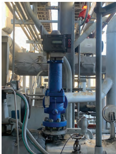
Wireless position monitor (left) is installed on one of the gas-compressor discharge headers; pressurized enclosure cabinet at right contains the wireless gateway and Modbus interface
