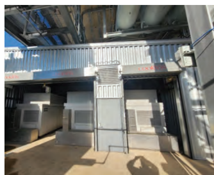
1. Temporary enclosure around compressors is at left, south side of finished enclosure at right
