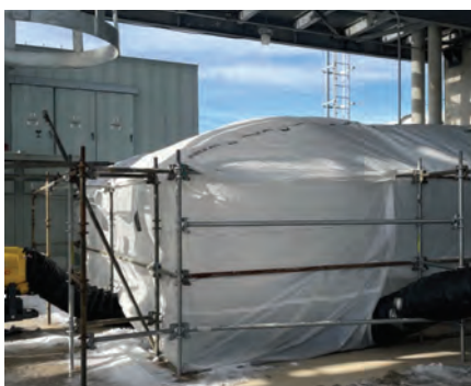
1. Temporary enclosure around compressors is at left, south side of finished enclosure at right
