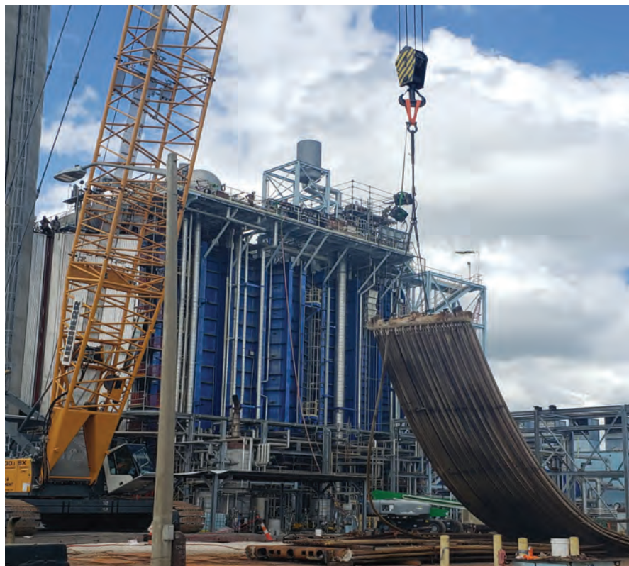
3. Harp sagging when a strongback is not used
