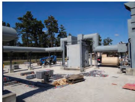
2. Circular non-seg bus runs from the generator (extreme right) to the circuit breaker in the generator accessory cabinet at the center of the left-hand photo; it is shown entering the generator step-up transformer in the right-hand photo
