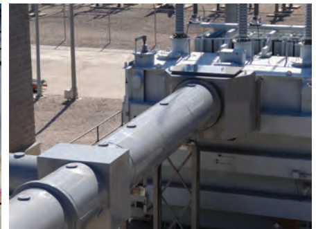
2. Circular non-seg bus runs from the generator (extreme right) to the circuit breaker in the generator accessory cabinet at the center of the left-hand photo; it is shown entering the generator step-up transformer in the right-hand photo
