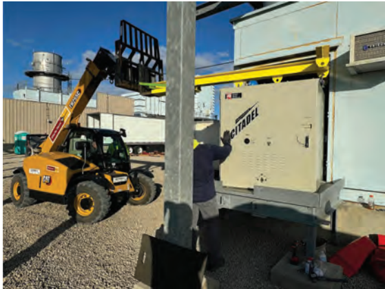
9. Citadel cell is lifted into the space formerly occupied by the original cell
