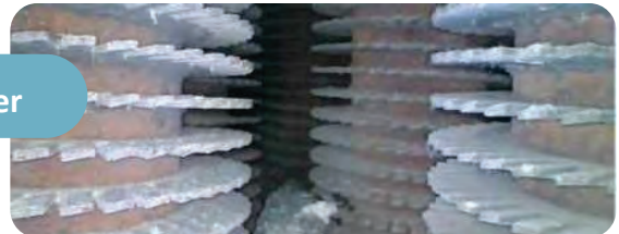
After cleaning 8th row of tubes
