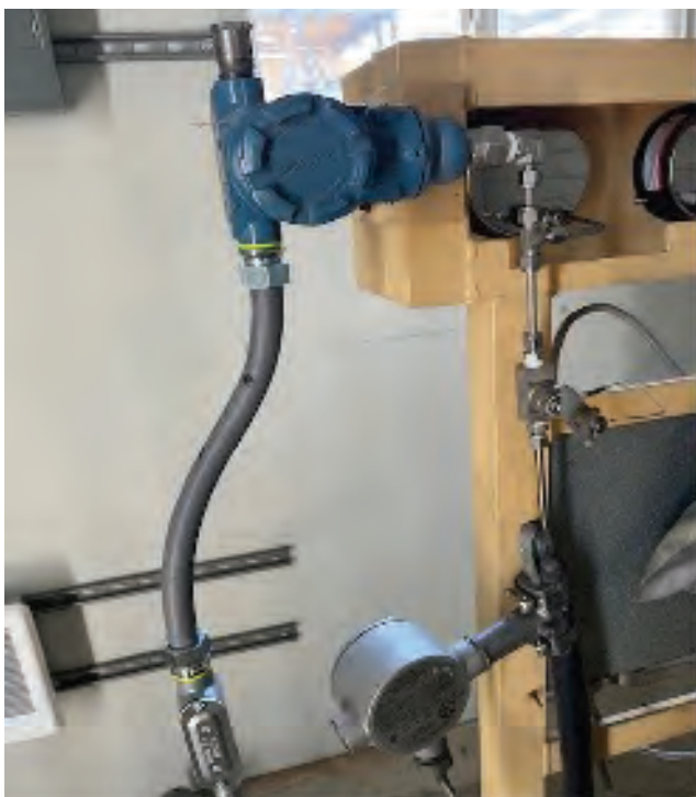
NOx-water pressure transmitter was relocated to protect against freeze-up
