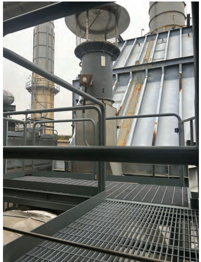
Ladder and work platform, a safety initiative, were mounted on the gas-turbine exhaust section (left). Platform provides direct access to the blower fan and motor for maintenance (right)
